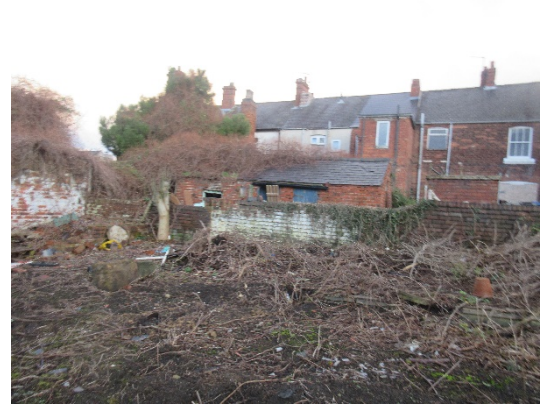
Photo taken from facing north east towards the rear elevation of Nos 25 and 27 High Street
